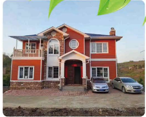
LIGHT STEEL FRAME VILLA 02
