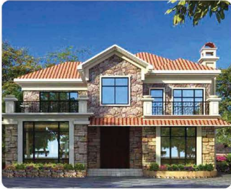
LIGHT STEEL FRAME VILLA 01
